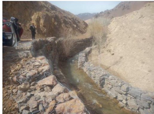
Figure 4: Gabion made at Yakawlang
